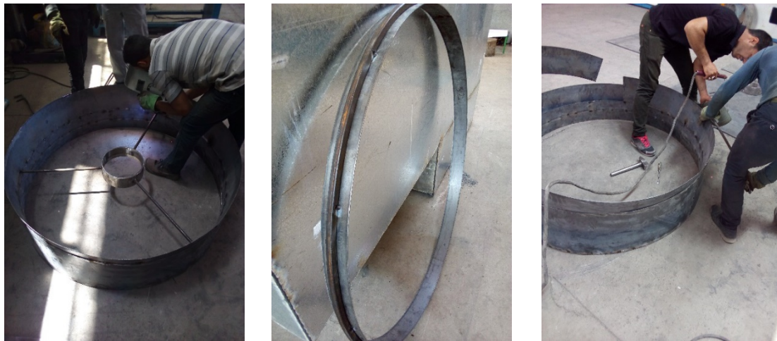
Figure 5. Duct fabrication process.
