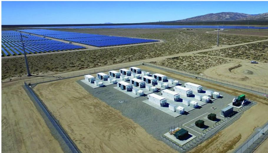
Figure 9. BESS co-located with PV plant
