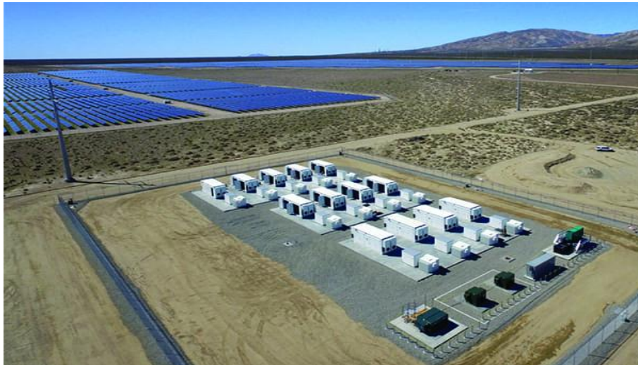
Figure 9. BESS co-located with PV plant
