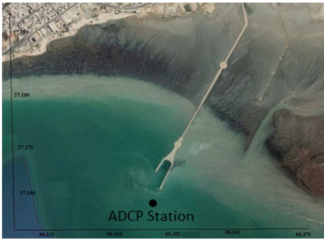
Figure 5. Position of field measurement of current and effective parameters and installation of ADCP device
