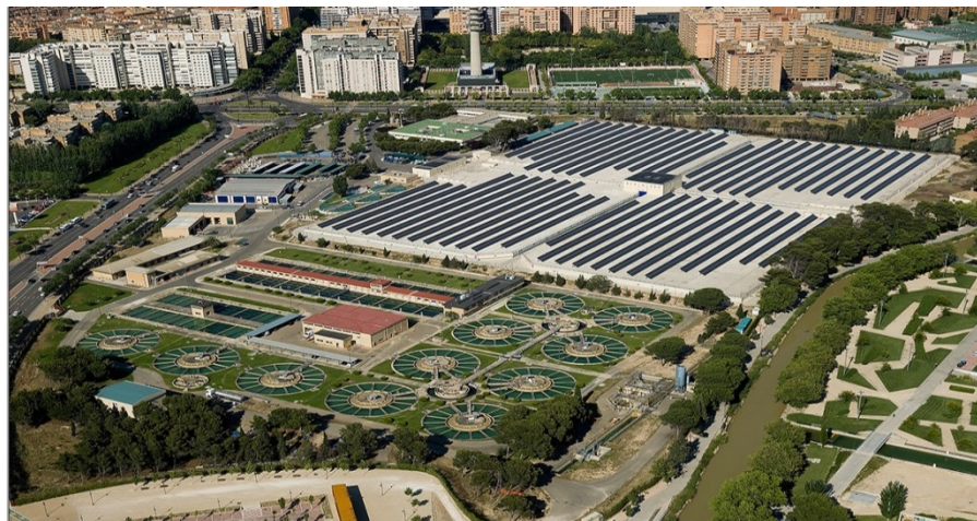
Figure 3. A water storage tank covered by solar photovoltaic panels [31]
