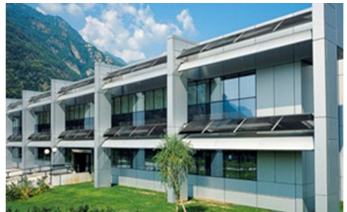
Figure 6. Inclined wall with windows
