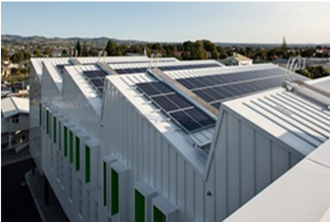
Figure 3. Saw-toothed north light roof
