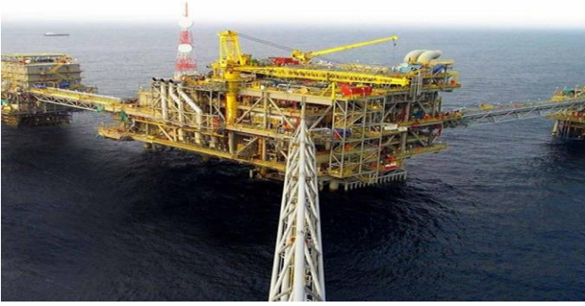
Figure 1. ExxonMobil offshore platform, Bonny Island, Nigeria.
