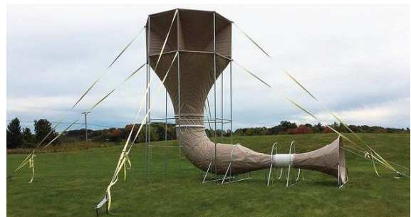
Figure 1. General outline of the INVELOX wind turbine system
